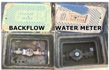
system is or could potentially be connected to any non-potable substance that could enter the public water system. When backflow conditions occur, pollutants or contaminants can enter the public potable water system through these unprotected connections.
