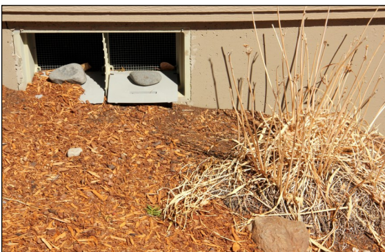
Above: approved bark is 18in. from home, with gravel Below: dangerous bark mulch is up against the home
