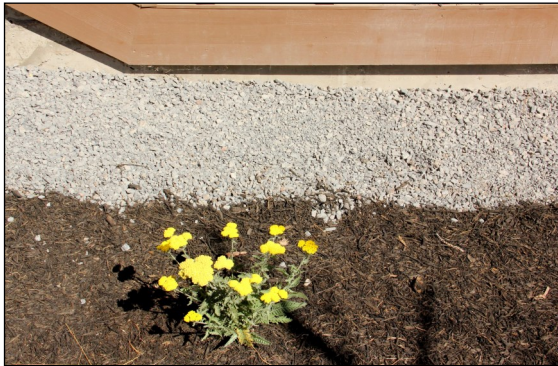
Above: approved bark is 18in. from home, with gravel Below: dangerous bark mulch is up against the home
